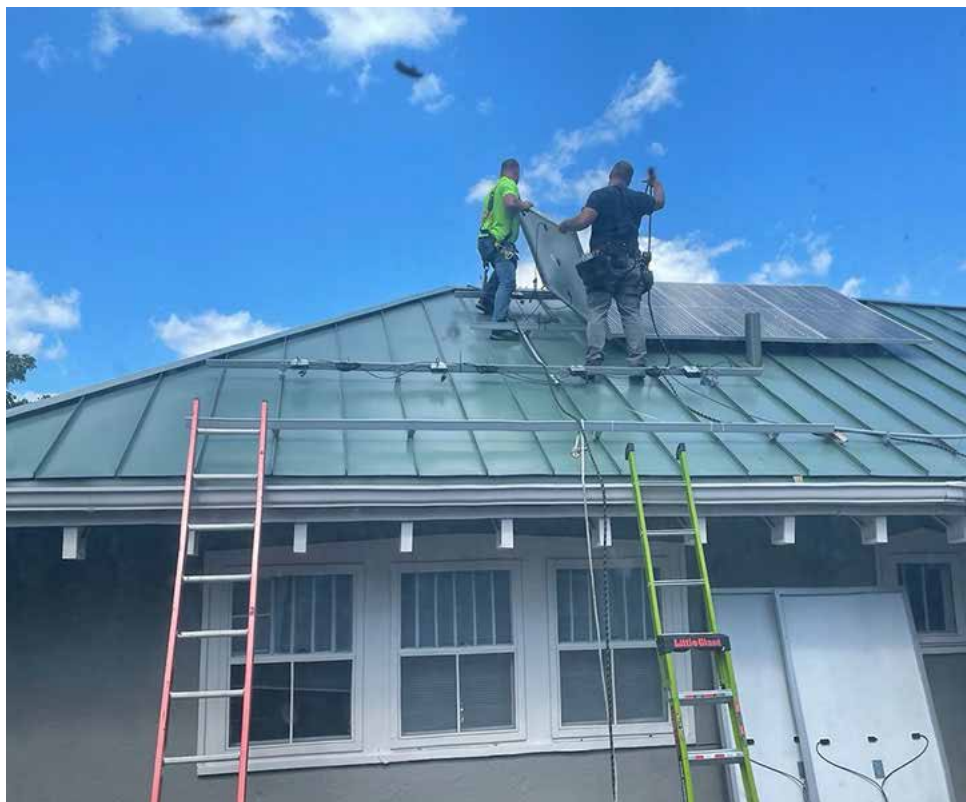
Installation of the solar panels in progress at the author's house
